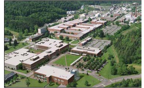
ORNL is located in Oak Ridge, Tennessee
